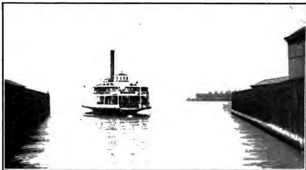
FERRYBOAT BERKELEY ENTERING THE SLIP AT THE OAKLAND MOLE
